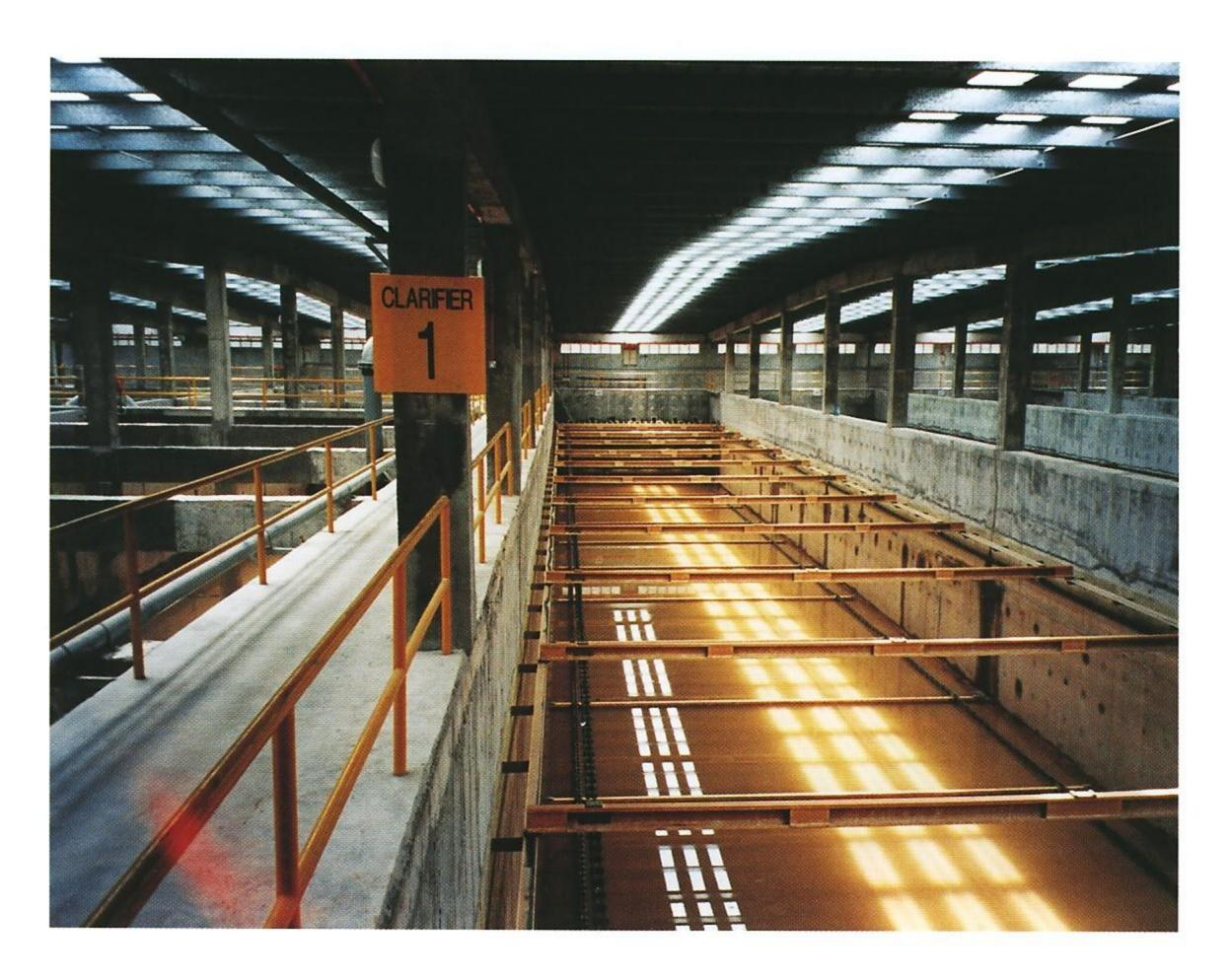
The Chain Scraper System For Effective Sludge Removal
